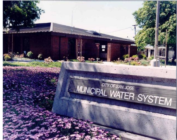
The Municipal Water System Building
